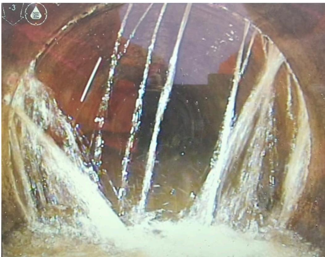
Monxton High Street - Groundwater entering the sewer via a pipe joint (July 2022)
