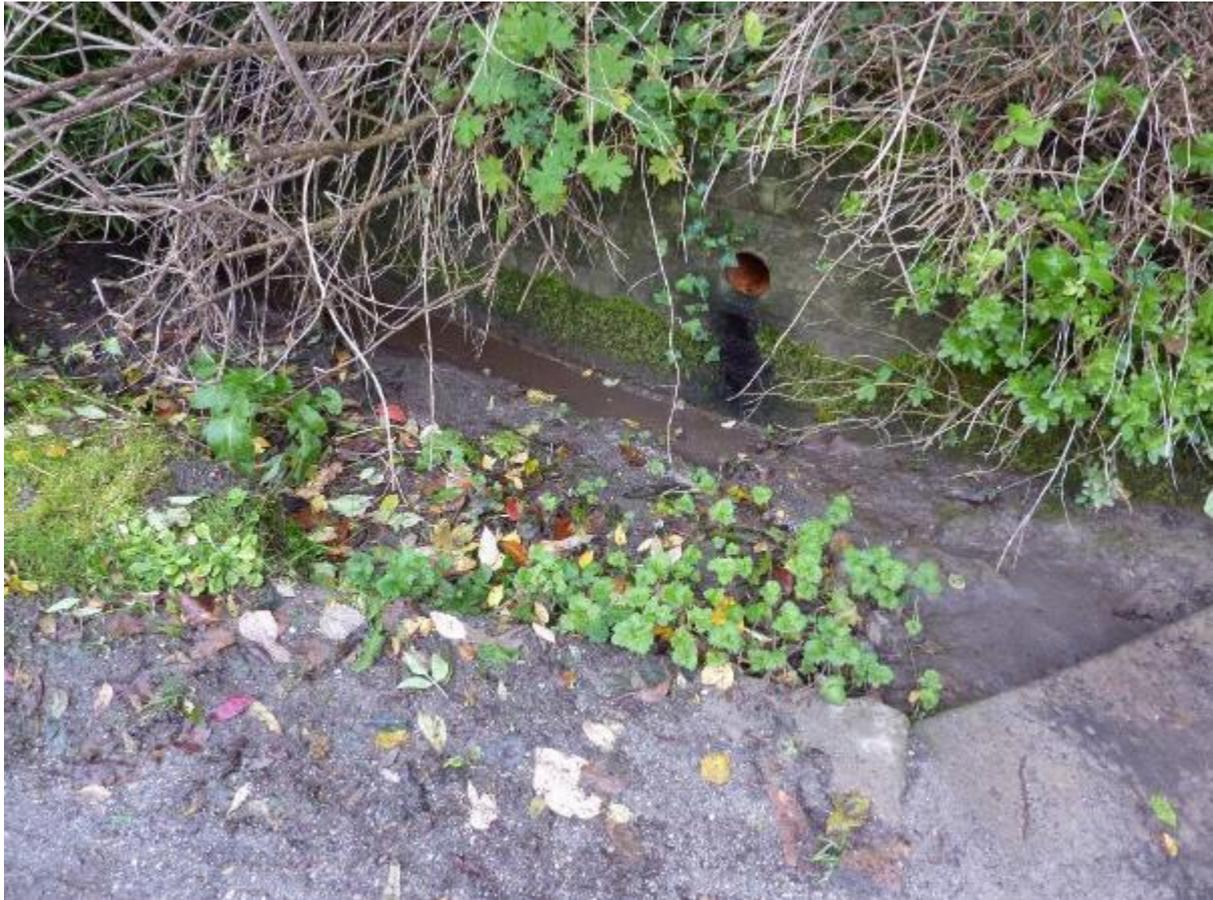
**Figure 4: Pollution pathways into the Cheselbourne: fine sediment and possible evidence of leaking heating oil**
