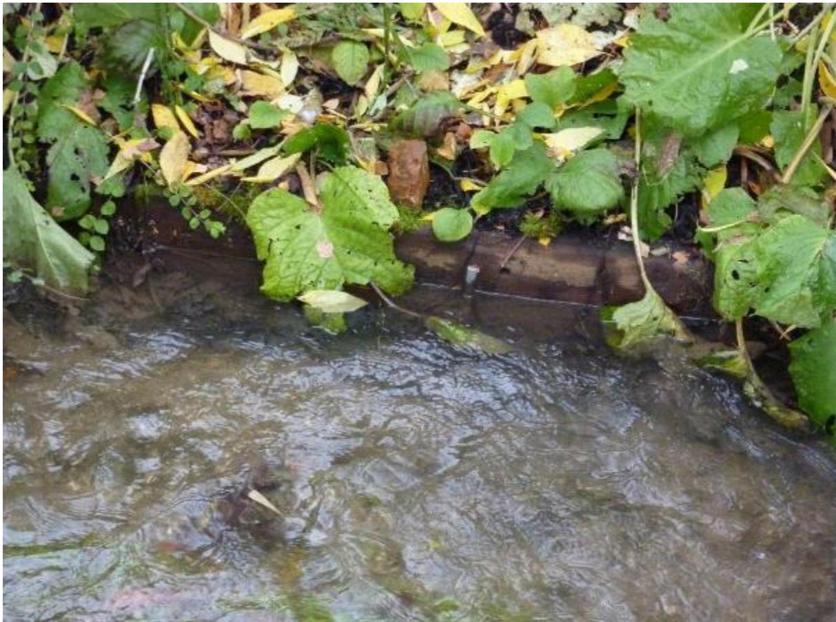
**Figure 8: Repurposed railway sleepers can be a significant source of long term chronic pollution as tar-based preservatives leach out into the stream**
