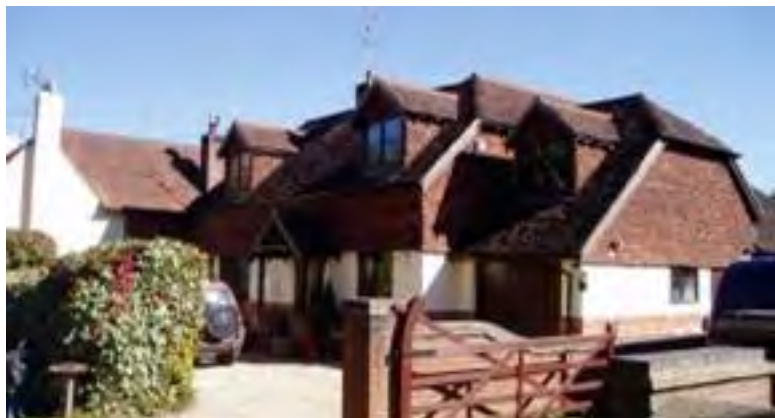
A new house built with old materials
