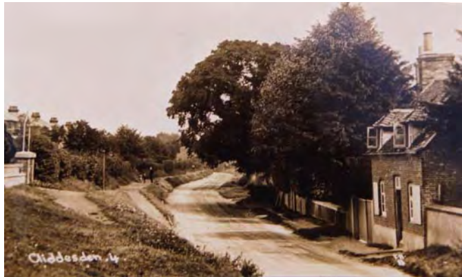
Looking North East along Farleigh Road with Farleigh Cottage on the right of the picture
