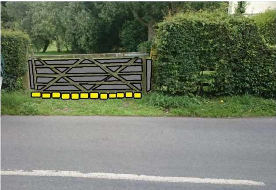
Image A – Field to north-west/upstream of Spring Hill Lodge. Barrier behind gate and alongside of Spring Hill Lodge on the right to hold water within field and prevent flow onto road.
