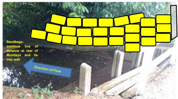
Image C – Immediately downstream of the Spring Hill driveway bridge, looking south west. Deploy either barrier or sandbags wrapped in polythene to raise river bank between bridge and the wall round Mundays
