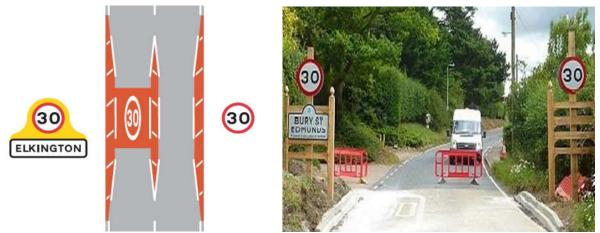
Figure 5 – Examples of speed limit gateway treatments
