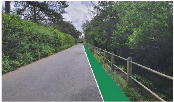
Figure 15 – Example of virtual footway along B3046 to protect pedestrians
