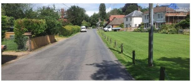
Figure 14 – Existing layout of B3046 and example with no centre line
