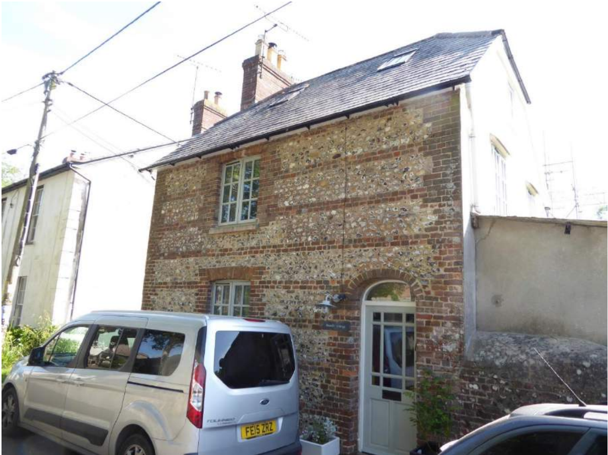
Figure 31: The use of flint and brick banding to walls
