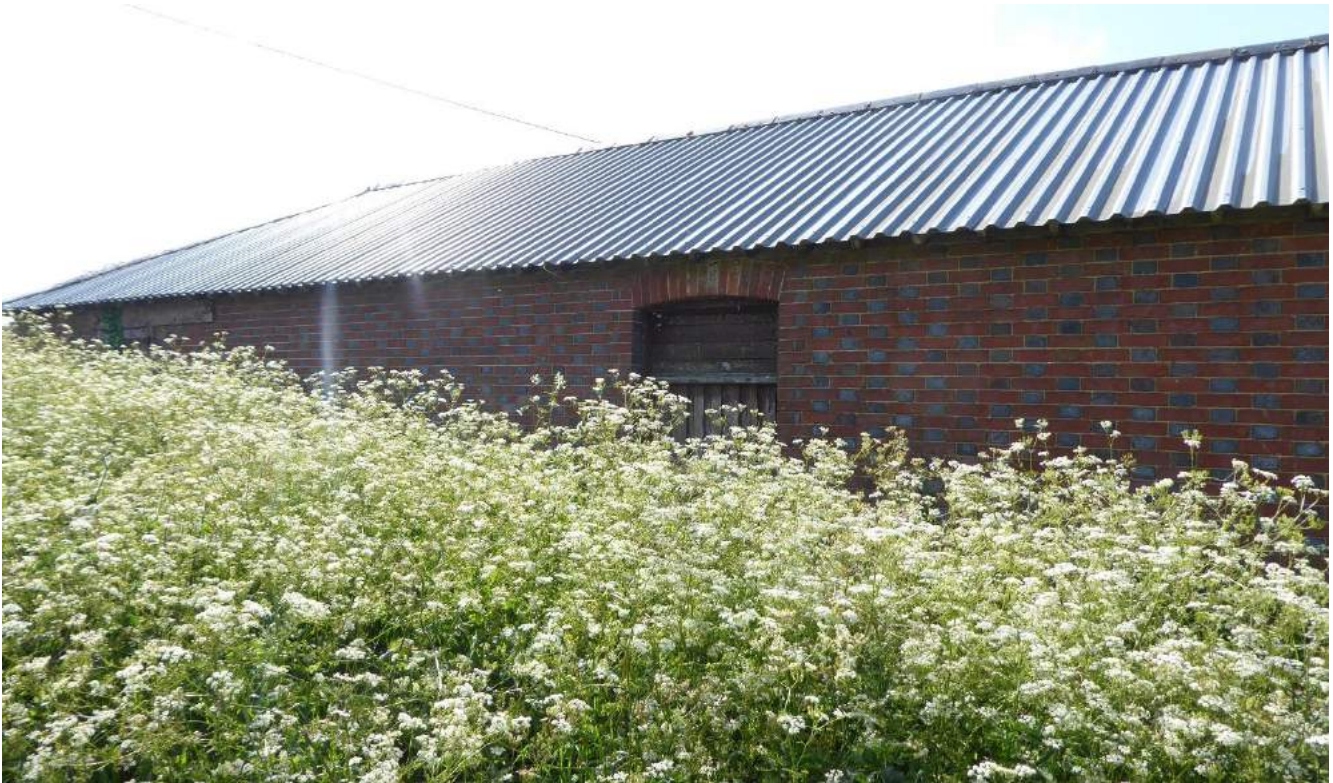
Figure 22: Manor Farm - Flemish bond with headers brought out in grey
