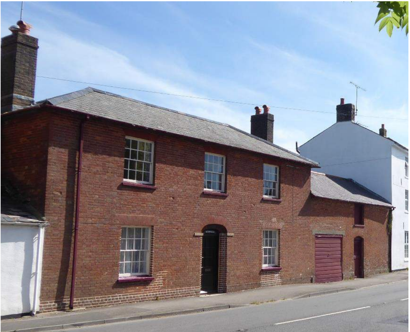
Figure 27: The use of segmental arches or flat gauged arches
