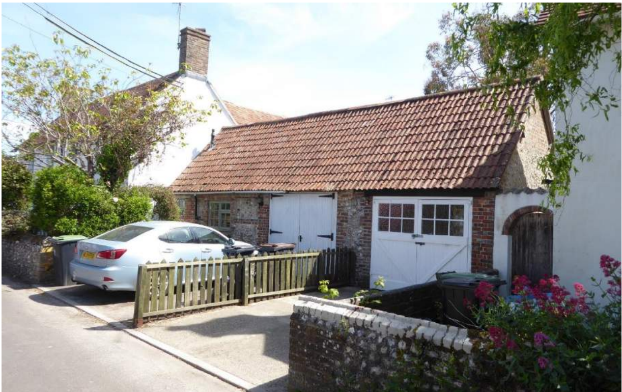
Figure 12: Bridgewater pantile, outbuildings to Chapel Street
