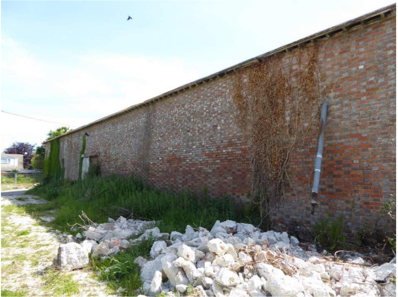
Figure 32: Flared headers used in Flemish bond to Manor Farm group
