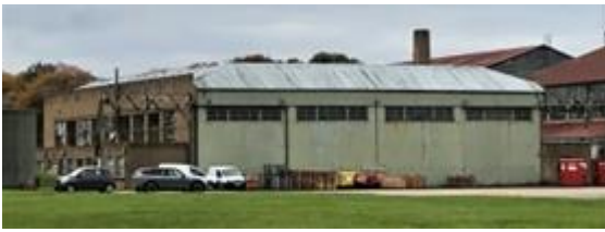
Hangar 4. A very unusual, scaled-down version of a 'C' Type Hangar showing the armour-plated doors on the northeast elevation.
