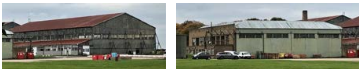
Left: Hangar 3 is one of two Admiralty 'F' Type Seaplane Sheds completed in 1922 and still in use today. Right: Hangar 4 is a very unusual, scaled-down version of a 'C' Type Hangar showing the armour-plated doors on the northeast elevation. Hard standing can be seen in front of both hangars.
