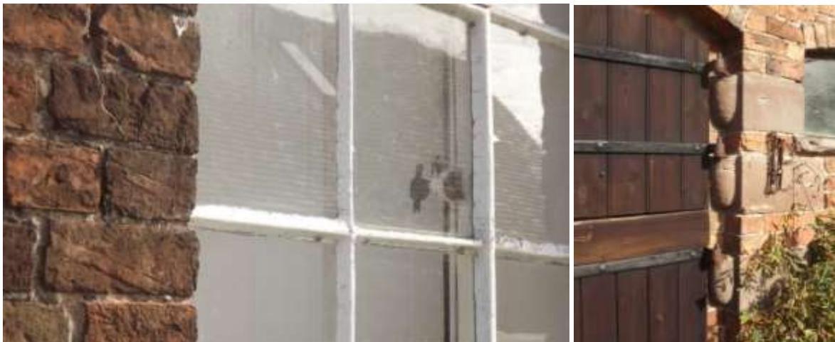
**Figure 9** Cast iron 'hand' window catches and moulded stone door hinge holders
