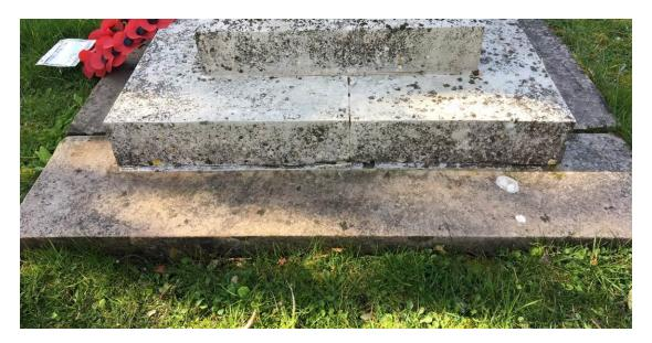
Fig.2 Detail of paving showing movement from tiered base.
