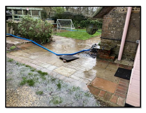
Fig. 2 Thatch End Foul Drain Propped Open to Take River Flooding
