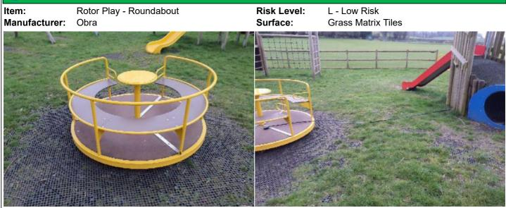
**Finding:** The falling space overlaps the free space between **Action:** Monitor - No remedial work recommended the embankment slide/crawling tunnel and the roundabout in contravention of the requirements of BS EN 1176:2017 Part 1
