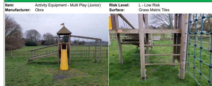
**Finding:** There are openings leading from platforms in excess of 1.0m in height to steep play elements and no hand supports complying with grip or grasp are provided, in contravention of BS EN 1176 Part 1: 4.2.9.4
