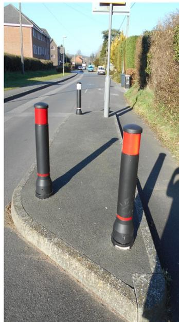
Figure 17: showing pinch point construction and the two wheeler/pedestrian lane
