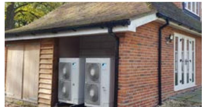
Figure 59: Place pumps in a recessed space to minimise the visual impact
