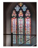
some glass is missing and the lead cames are bent. What's more, the whole light is distorted so the plan is to remove it, relead it and replace the missing pieces with newly painted quarries to match. Fortunately, the Friends of Kent Churches
