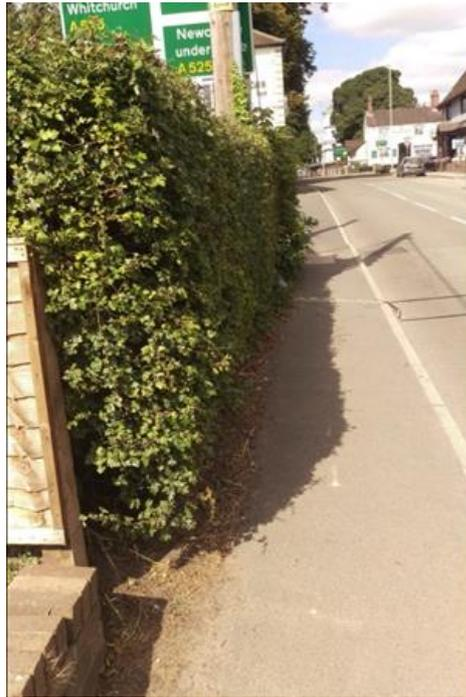
9.3.2 The hedge encroaches onto the footway restricting the usable width of the footway for pedestrians over this short section. This is an important length of footway taking into consideration the proximity to the school access and the understanding of the use of the Falcon car park for school drop-off and pick-ups.
