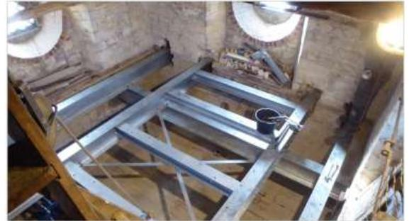
New steel girders span inside the tower, in the 'spare' storey below the old belfry
