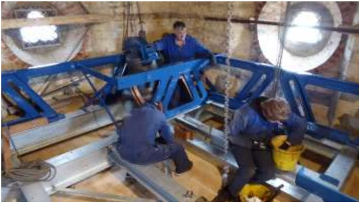
One benefit of the new bells being mounted lower in the tower, is that the ropes are shorter and less likely to stretch; this makes them more sensitive and easier to control by the ringers.
