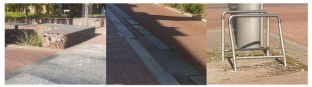
Repairs required to central brickwork, pavement edge and cycle racks to be replaced/removed
