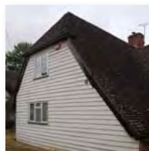
The Barn House weather boarding
