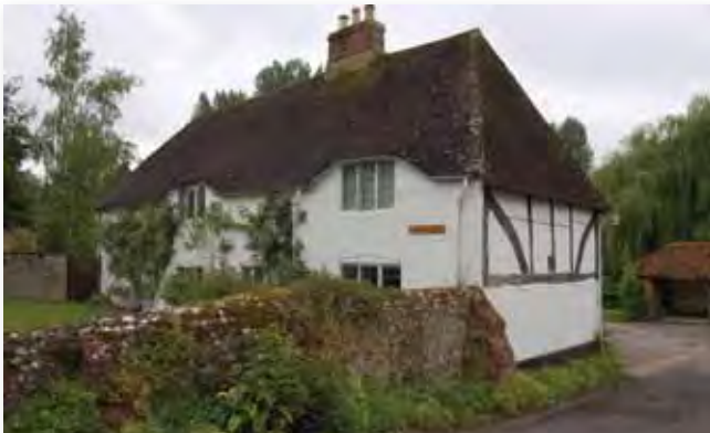
Haydown Farm House
