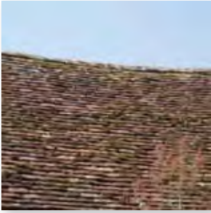
Place Farm roof tiles
