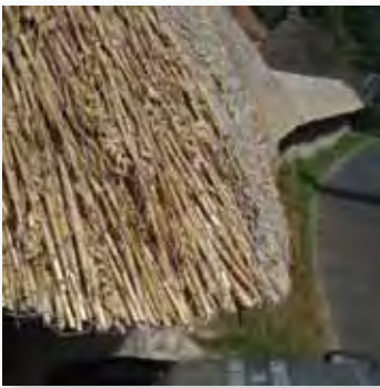
Detail of cob wall with thatched coping at Nether Wallop
