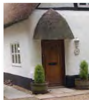
Brockhurst Cottage door detail
