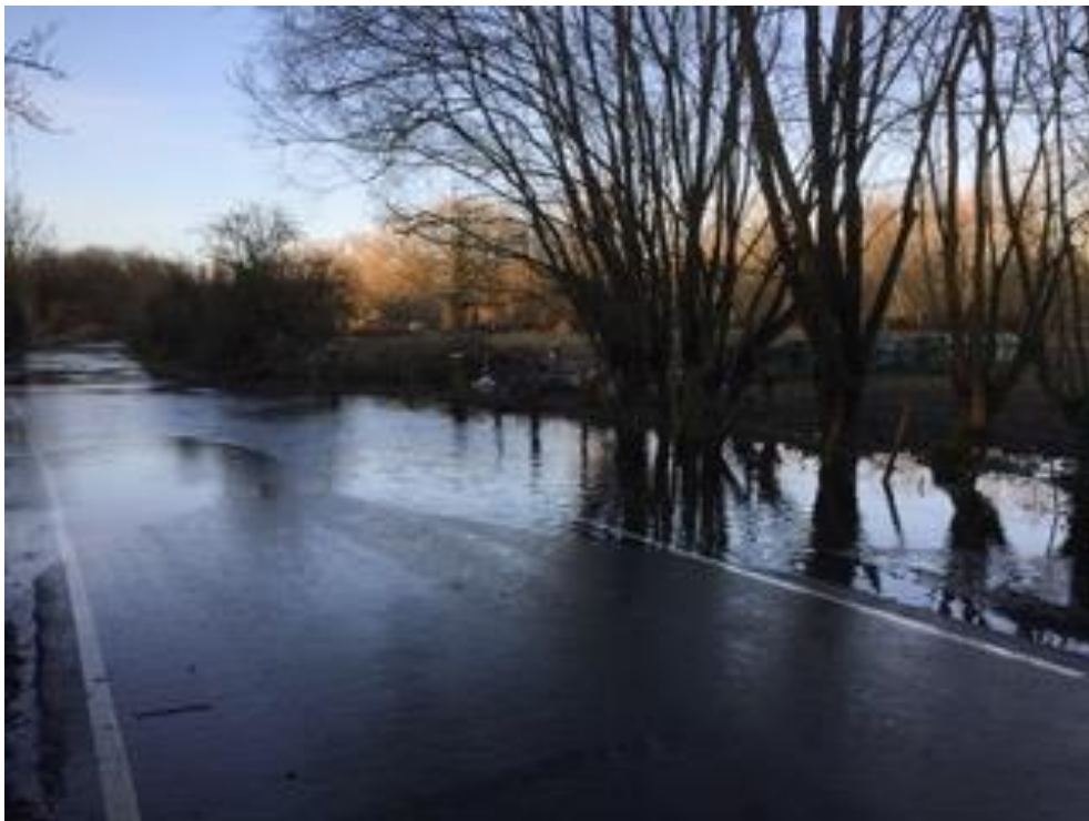
Flooding on Watery Lane
