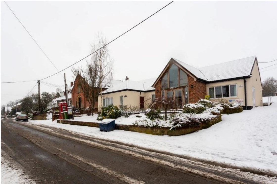
Upper Clatford Village Hall
