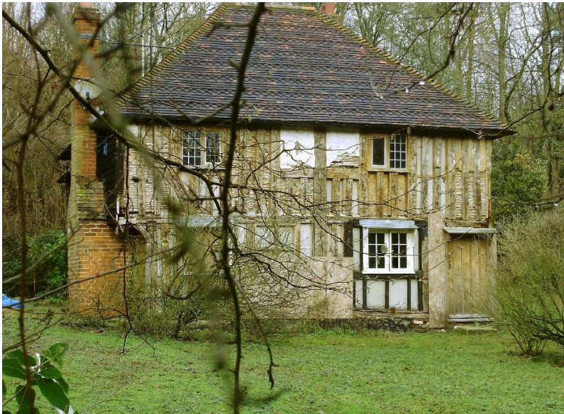
Plate 9. Left: Pett Dane (c.1500) abandoned and derelict, but now undergoing works.
