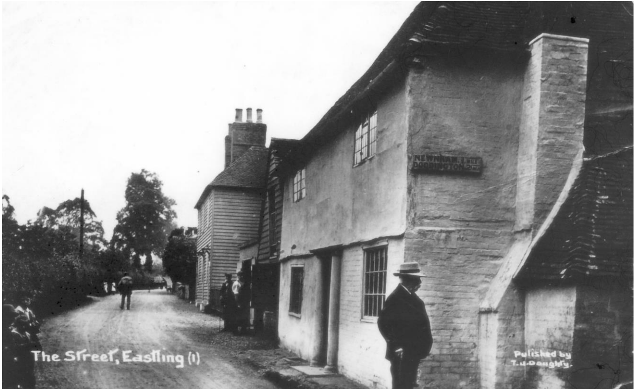
Plate 25 Above: Eastling Street from the corner with Newnham Lane. In the foreground the Old Forge with the saddler's shop behind. Photo published by Doughty's.
