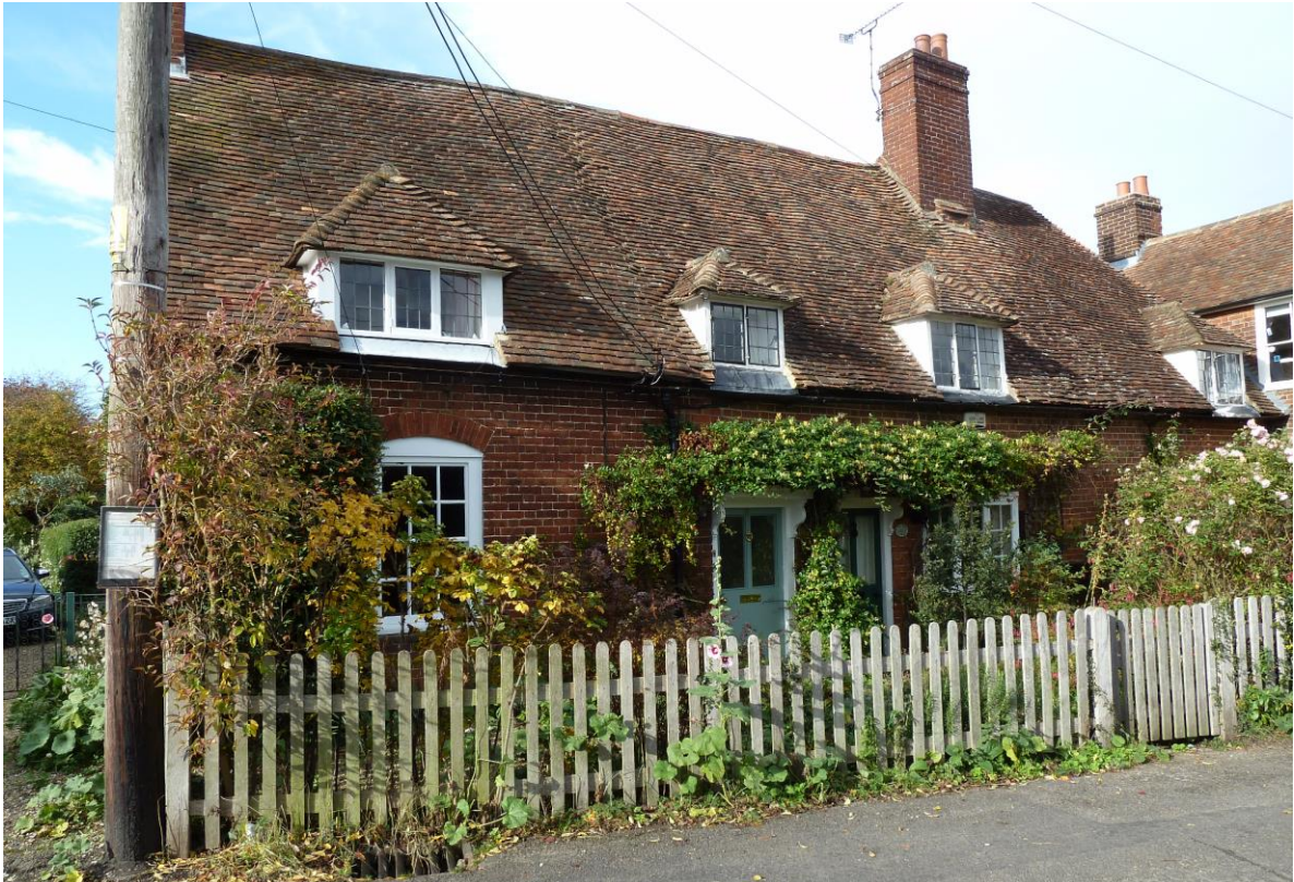
Plate 15. Above: Originally a single timber-framed building Number 2 is clad in brickwork, and Numbers 3 & 4 in hanging mathematical tiles
