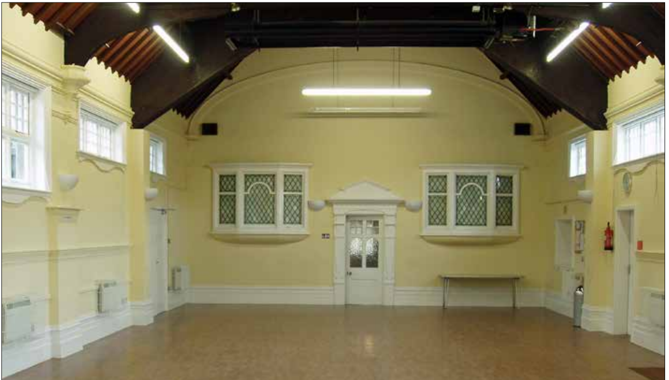
Fig 4.8 Main hall after renovation showing new floor and hatch to kitchen in far right corner. Electric wall heaters were installed to provide heating at times when overhead gas heaters where too noisy to use.
