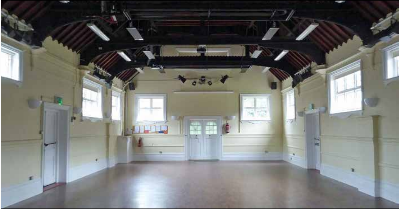
Fig 5.9 In August 2023 infra-red heaters were installed in the main hall replacing the electric wall heaters and the lower parts of the walls were repainted. Note too the low energy ceiling light fittings which were installed in 2015 replacing the old fluorescent tubes.
