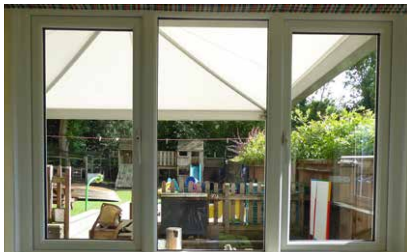
Fig 5.6 In 2021 The windows in the nursery were replaced with double glazed units.
