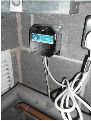
**Caltronic electronic scale inhibitor on the mains in boiler room**
