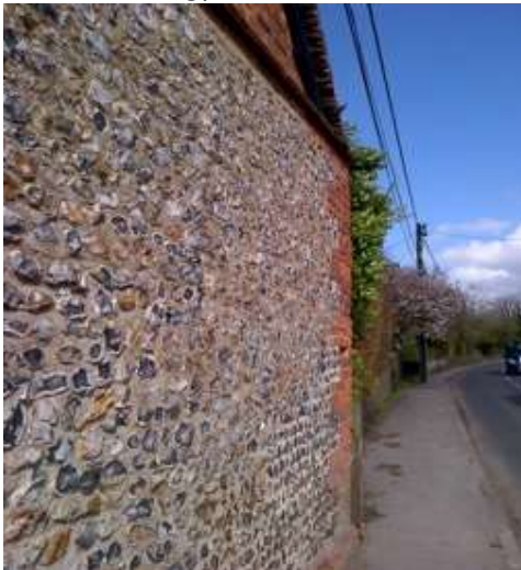
Figure 13 – Harcourt – knapped flint wall.
