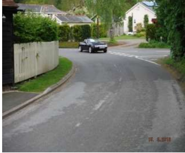
Figure 30 – poor visibility at corner junction of Stanbury Road and Village Street.
