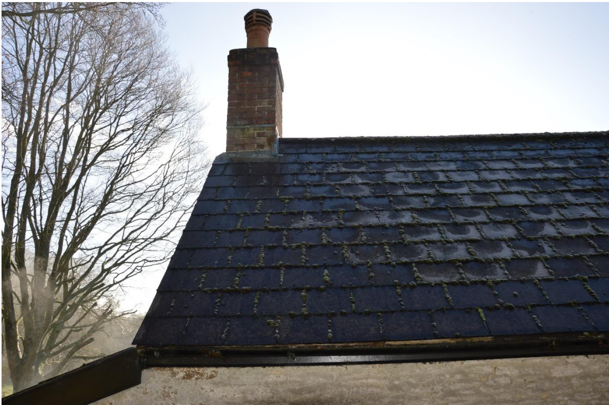
Plate 3. Tightly fitted slates and ridge tiles on the main cottage roof.
