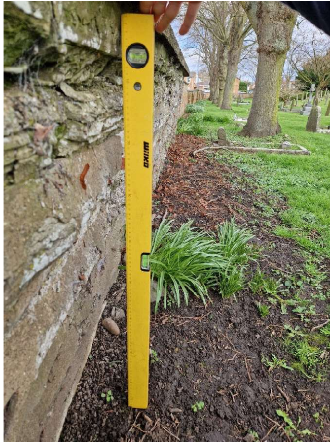
Photograph No. 7 – West – Lean to Rear Face of Wall
