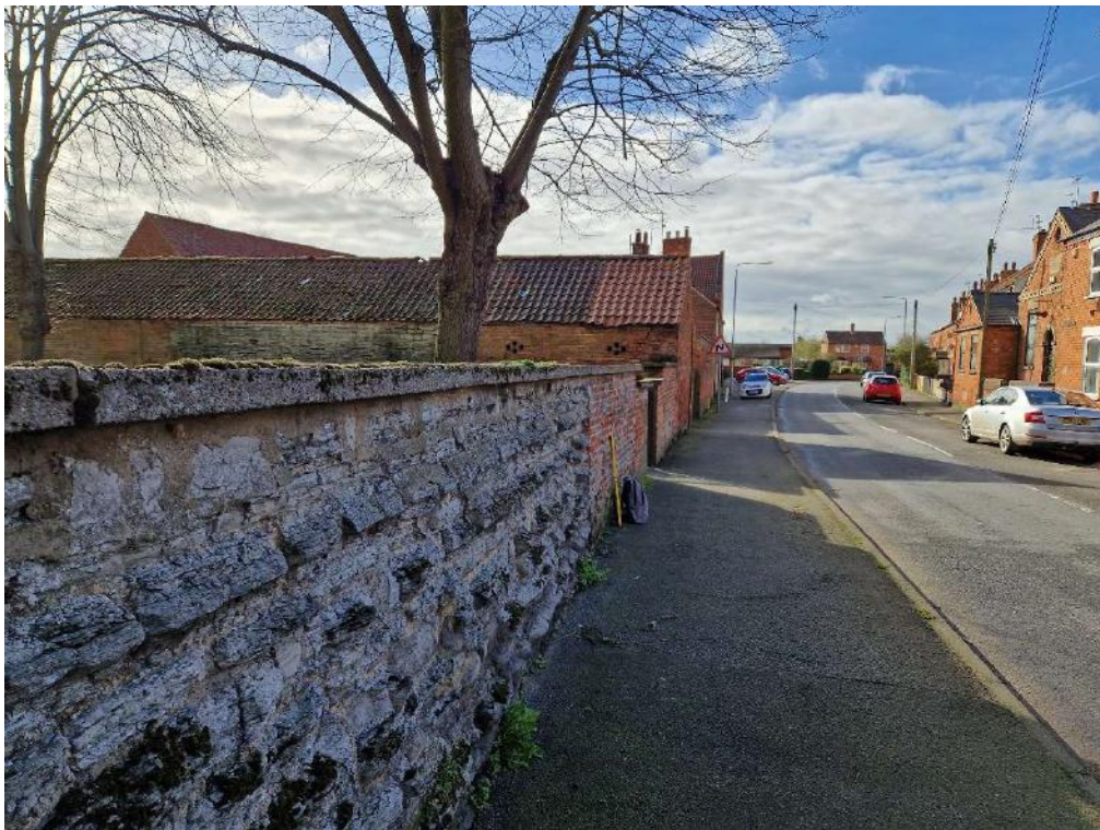
Photograph No. 2 – West – Spans 1-4 with Blue Lias Section in Foreground
