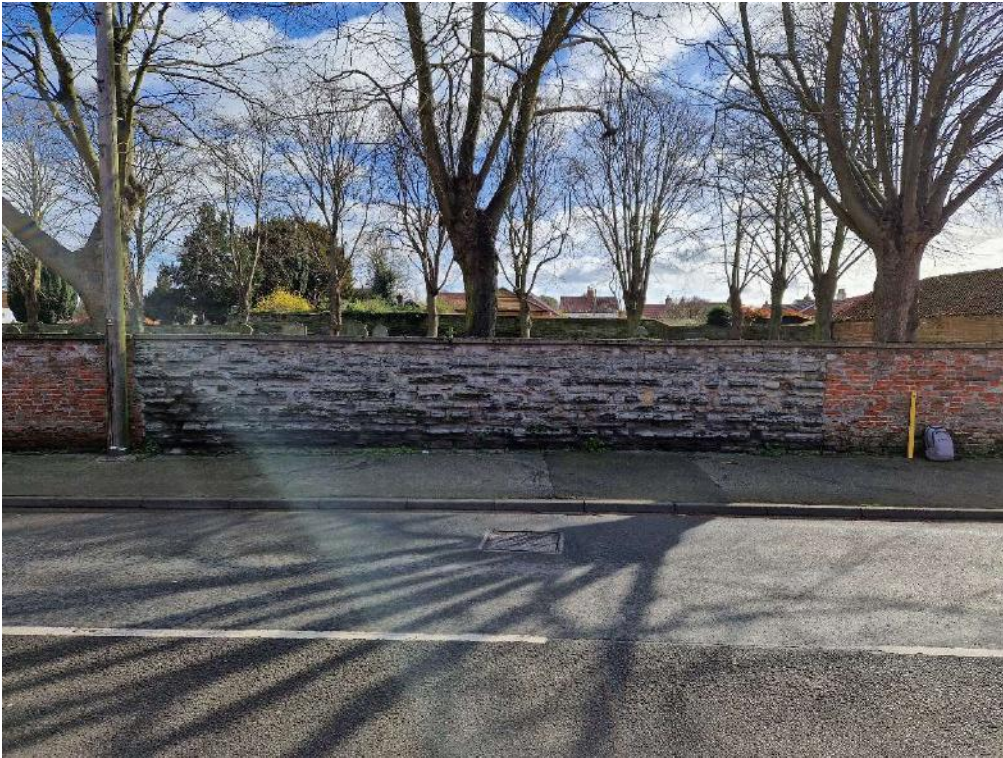
Photograph No. 3 – West – Span 4
