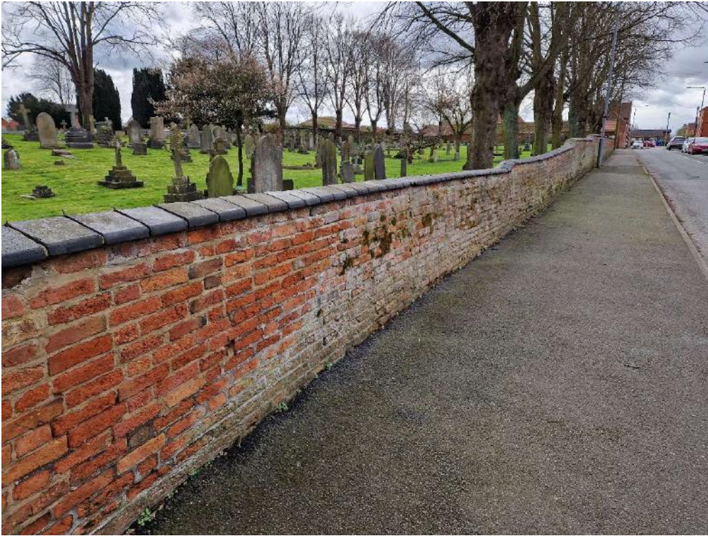
Photograph No. 15 – West – Span 7
