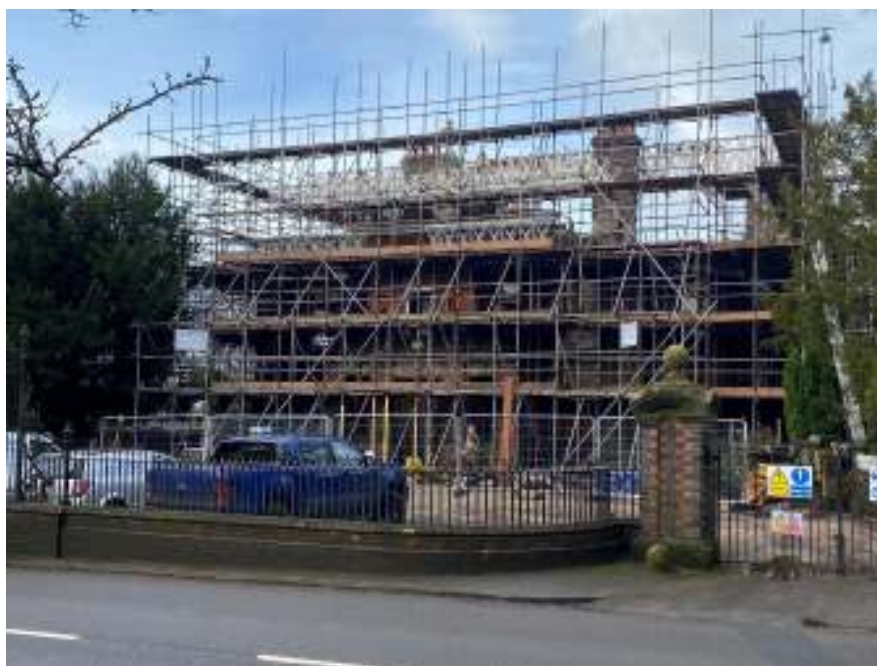
Betley Court scaffolding, January 2021
