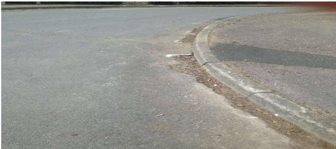
Gutters were weeded and brushed
