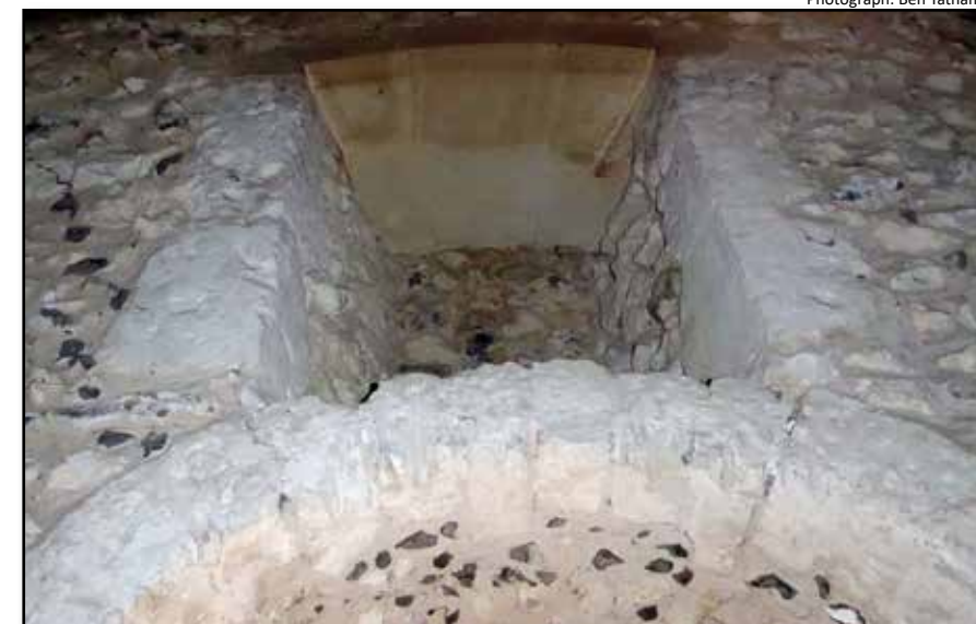
Blocked-up Saxon window on inside west wall of church tower. The white stone is rock chalk, probably from the mine in Westhumble (now the bat caves)
