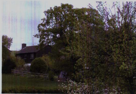
The angularity of the building breaking the skyline clashes with the natural shape of the landscape
