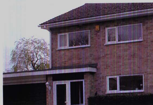
A shallow pitch, concrete tiles and sand faced bricks detract from individuality
