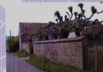
A traditional, well considered garden wall
