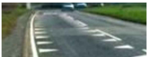
DETAIL 7 AN EXAMPLE OF DRAGONS TEETH LEADING TO FAKE SPEED BUMPS AT ENTRY TO VILLAGE AT SOUTH END
