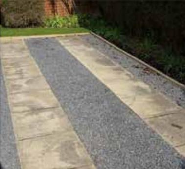
Driveways that are a combination of hard-paving and gravel/grass allow for drainage, whilst also remaining a suitable area to drive and walk on.
