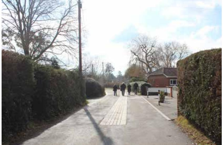
Central drainage channel to a road allows for the edges to be used by pedestrians and cyclists without obstruction.
