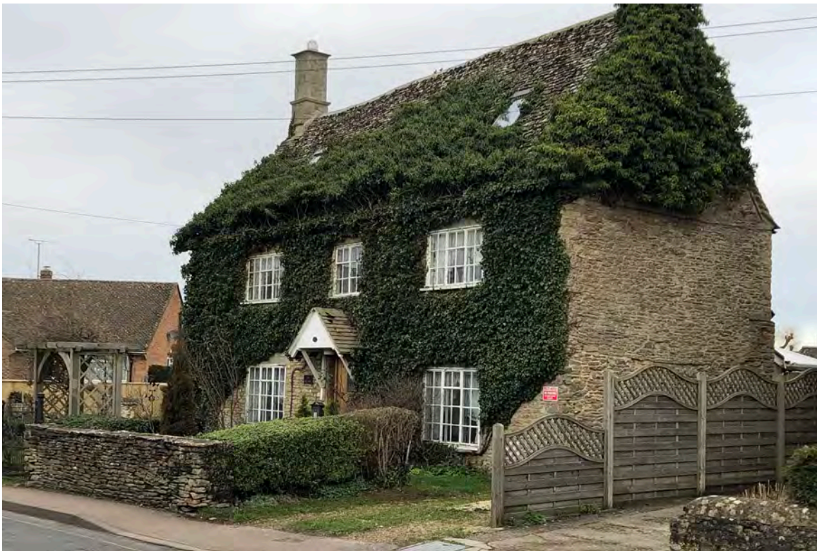
Squires Cottage, 11 Station Road
