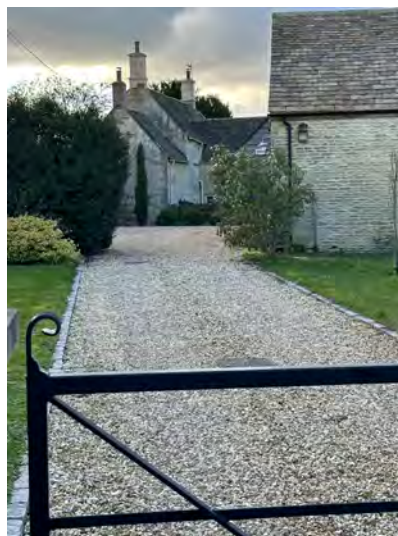
Yew Tree Cottage (60 Station Road, Listed)
