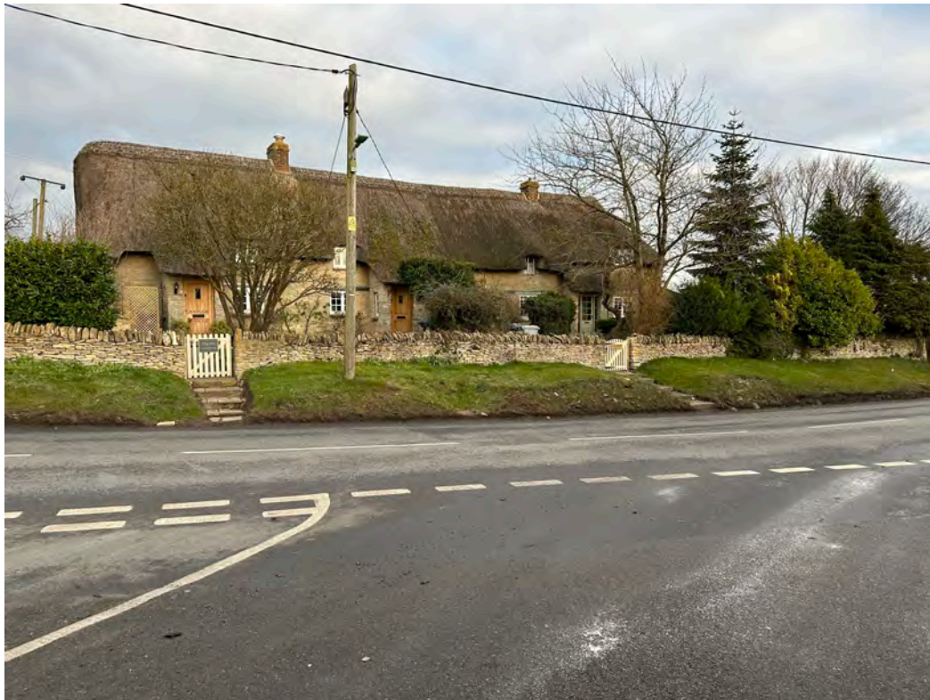
Pilgrim Cottage and Chapel Hill Cottage, Manor Road
