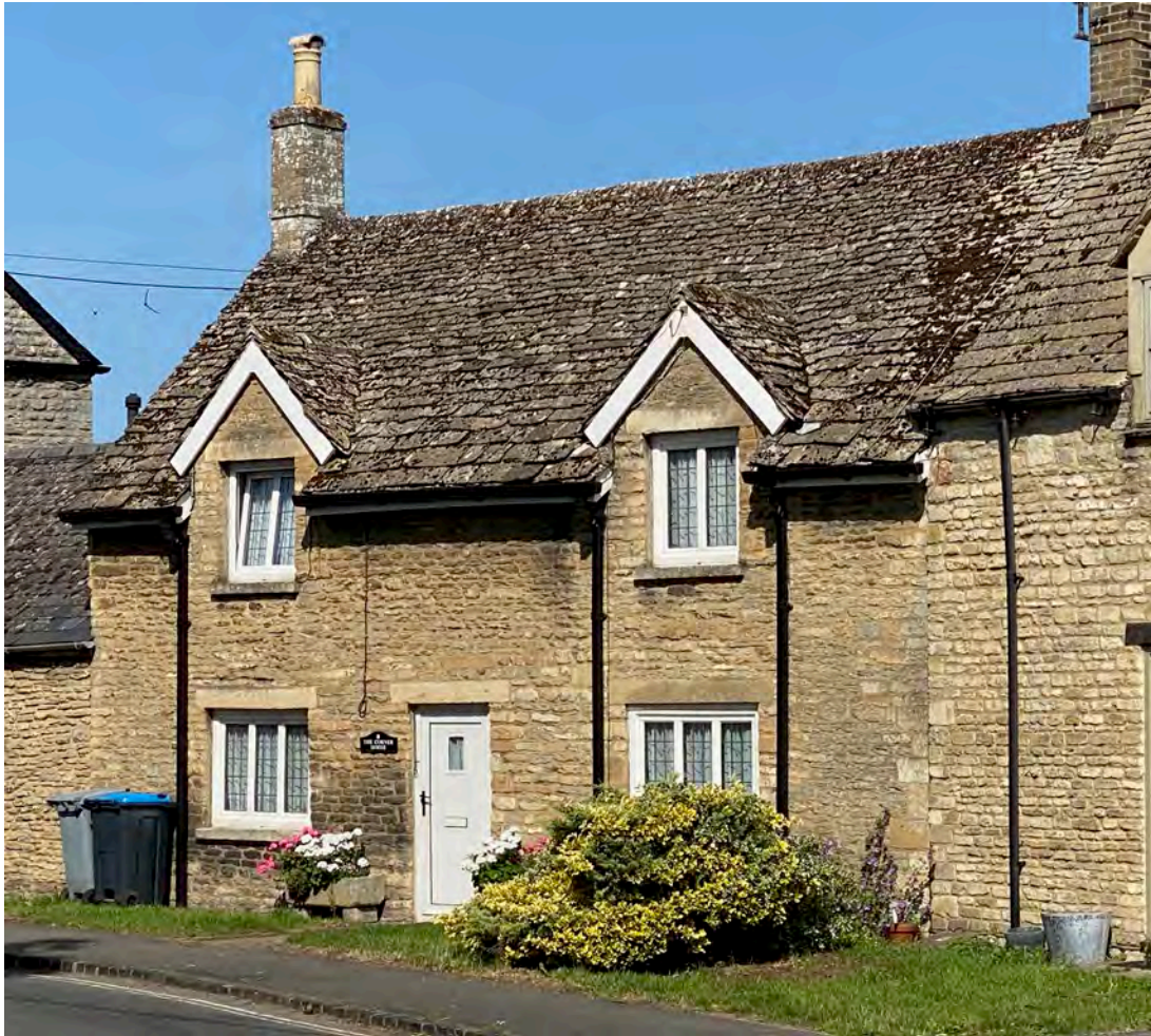
The Corner House – Carterton Road
