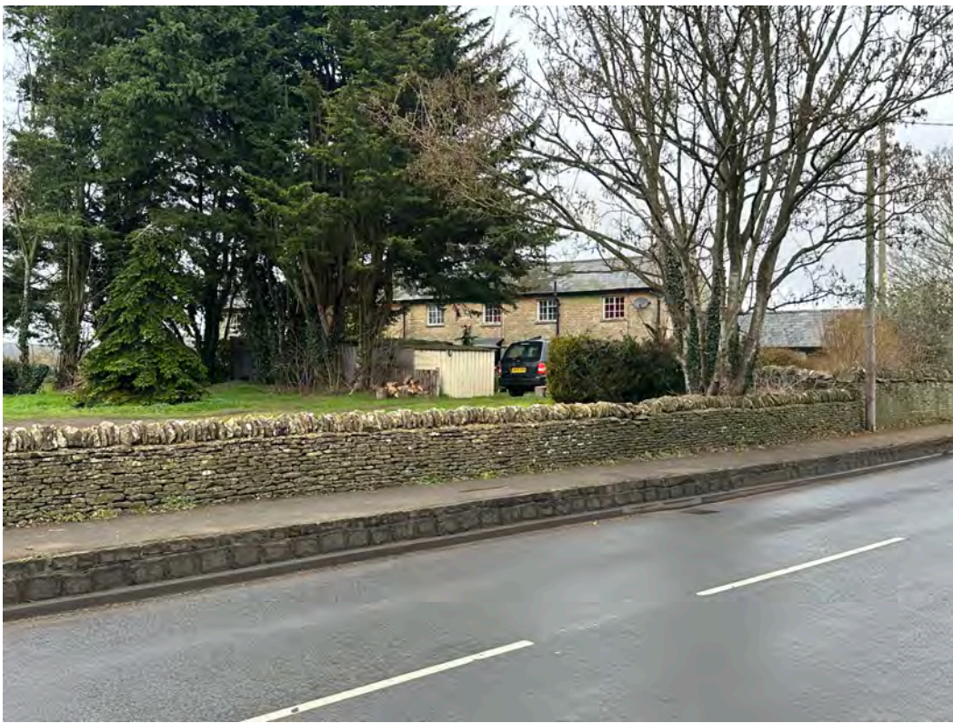
Front Elevation of Nos 1 & 2 Manor Farm Cottages. Manor Road
