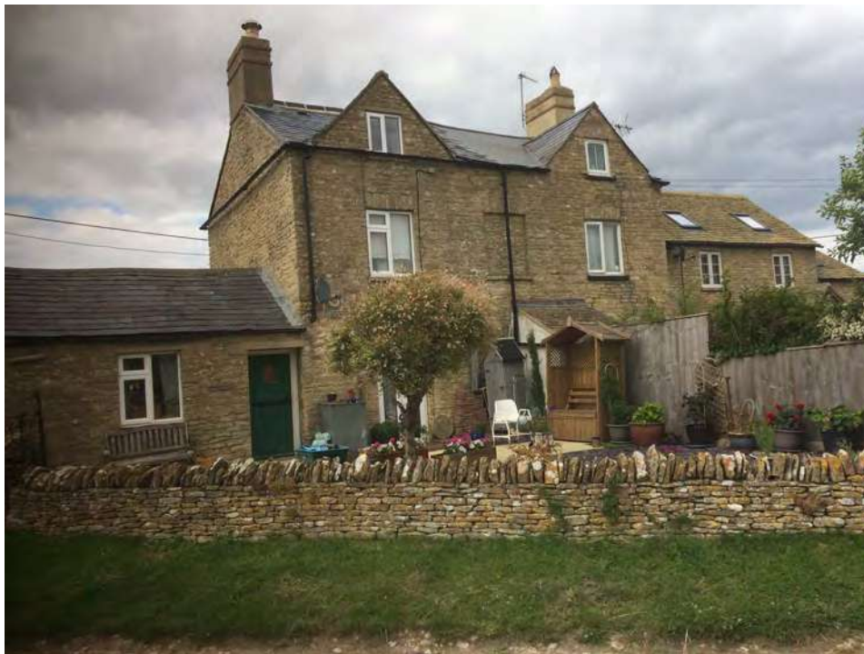
Fennel & Richards Cottages, Chapel Hill
