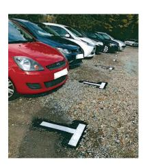
The Town Council are pleased to report that essential repairs and improvements to the overflow car park in Mount Street are complete. Thermoplastic lining has been applied to identify designated parking bays, which, it is hoped, will allow free movement around the car park and prevent vehicles being blocked in. Users are requested to park only within the marked bays.
