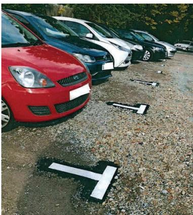
The Town Council are pleased to report that essential repairs and improvements to the overflow car park in Mount Street are complete. Thermoplastic lining has been applied to identify designated parking bays, which, it is hoped, will allow free movement around the car park and prevent vehicles being blocked in. Users are requested to park only within the marked bays.
