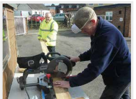
Mark cuts the timber to length with Keith.
