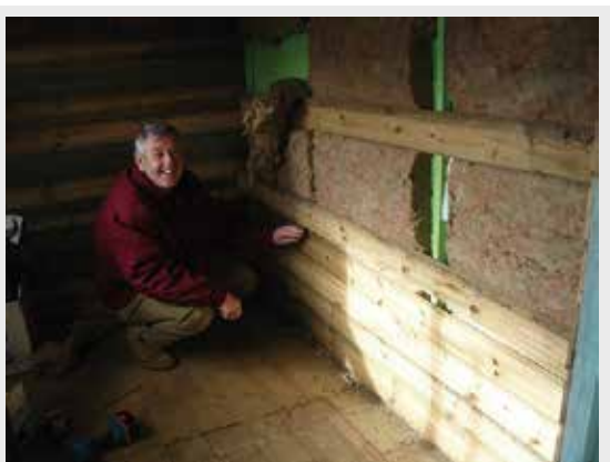
23 Feb. David sorts out the inner wall.
