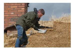
To increase the angle and improve water run off, after all that's the point of the roof, the top of the ridge is raised. It has a thick central roll of water reed with bundles of combed wheat straw bent over it, once again held down by hazel – long straight pieces called liggers, with shorter ones forming the diagonal pattern, all held down with more bent hazel spars.
