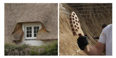
The top of the coat or OVERSAIL (the part that gives the roof-in-progress a punk mohican look) has to be trimmed off. Then long rolls of reed are placed along the apex of the roof to SET THE SKYLINE, evening out any irregularities and ensure the ridge has a steep pitch
