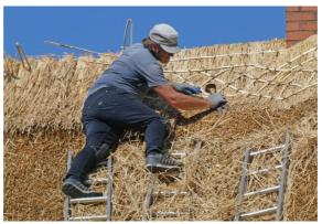
There are 2 main types of ridge and Ladbroke has examples of both. *Church Cottage* and *Attwood Cottage* have a raised ridge with a patterned cut edge while *Sarah's Cottage* and now *The Cottage* have the more traditional flush ridge. To make this, the bottom of the ridge is cut off with a thatcher's scythe and then manicured with shears so it appears to flow seamlessly into the main coat.
