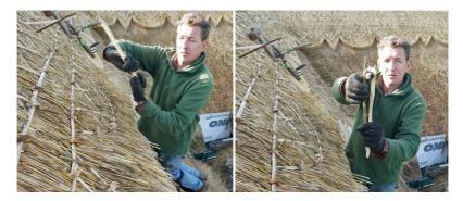
The ridge pattern is roughly cut with a knife and large shears and then fine-tuned with manicure scissors, well it looked like that from the ground but close to I could see they were small topiary shears. Church Cottage's ridge has a traditional *points and scallops* pattern and once a section is finished wire netting is fixed over the thatch to protect from hungry beaks and mouths.
