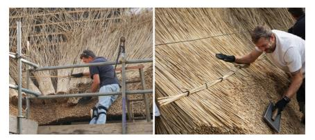
Finer detailing of the base of the reed, eg near dormer windows, is created using a narrower wooden bat called a DUTCHMAN. Once the reeds are in the correct position they are fixed using a thin steel sway. Layer upon layer is built n this way.
