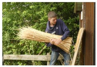
Preparation is key to a good finish. First of all the top layer of the old thatch is removed and any irregularities evened out, otherwise the top surface would look lumpy (anyone putting roll-out icing over a rough cake surface will know what I mean). It's also critical and very laborious to get the straw flat and even. Each sheaf is split into
