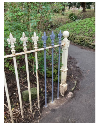
Replacement railings ready for painting
