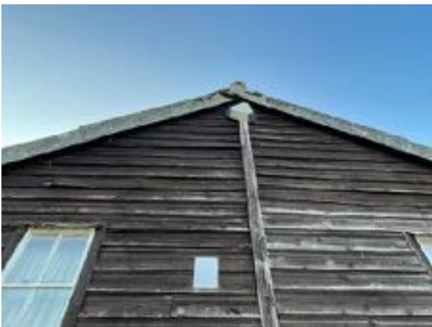
Figure 9 - Gaps between wooden panels SE elevation
