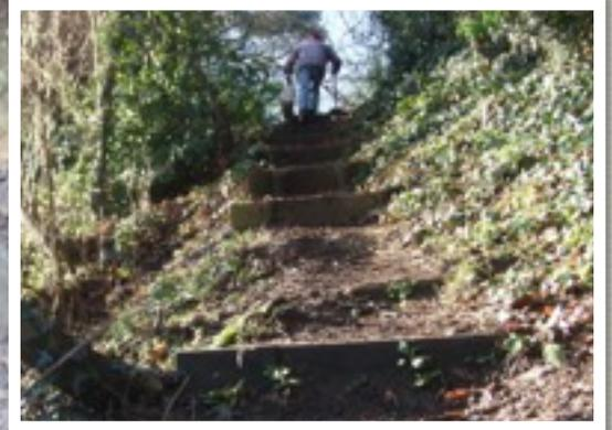
TOO DEEP, UNEVEN TREAD AND SOME IN NEED OF A HAND RAIL. BETTER DRAINAGE ON THE STEPS IS BADLY NEEDED. THIS MUDDY MESS IS NOT GOOD ENOUGH.
