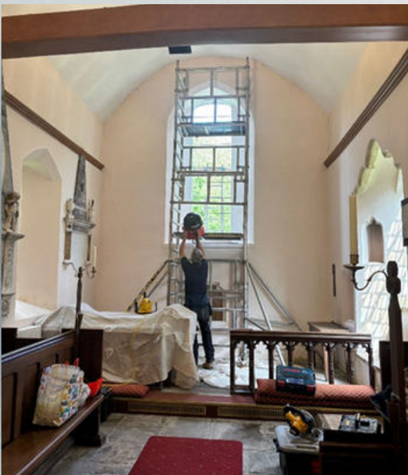
Restoration team at work
