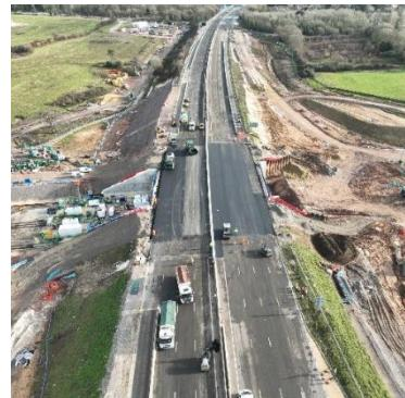
The closure, which began on Christmas Eve, allowed engineers to install a new underpass at Junction 10 using an innovative "box-slide" technique — only used a handful of times in the UK. A 60-metre pre-built concrete structure, weighing around 8,500 tonnes, was slid into position before the motorway surface was reinstated. This approach avoided months of lane restrictions and overnight works.
