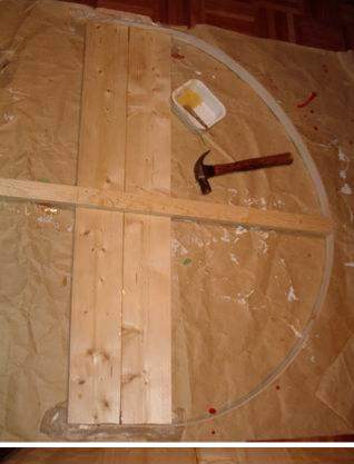
Two plywood laths are wrapper around the ends of the seat and the lengthwise batten. This is the first, innermost layer of the gunwale. The laths are cut to such lengths, that the ends land on the ends of the seat.
