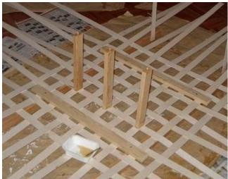
Three vertical supports are glued and screwed under the seat. Supports can be round or square, 1" to  $1 \frac{1}{2}$ " in diameter, and made of some light wood. The length of the supports is 12" (30 cm).
