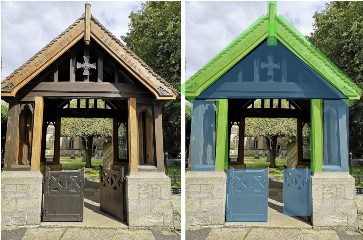
Image 1: Lychgate, front elevation: showing external surfaces within Scope of Works
