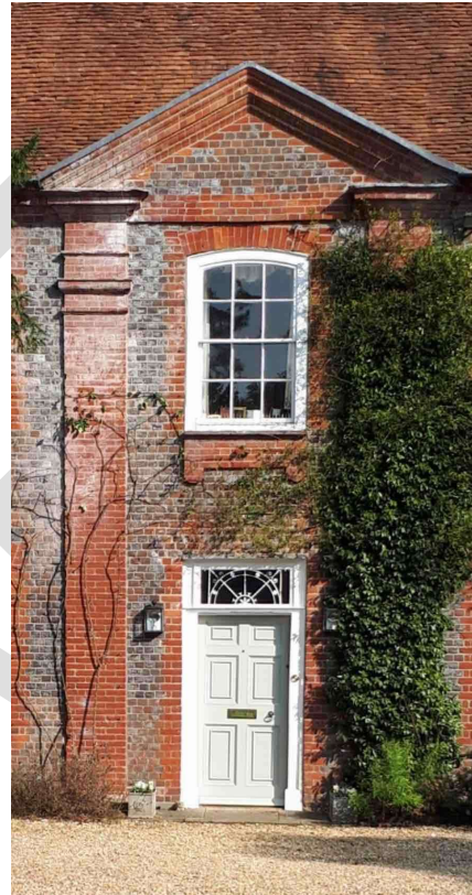
Figure 29: The Old Vicarage, features of the south elevation
