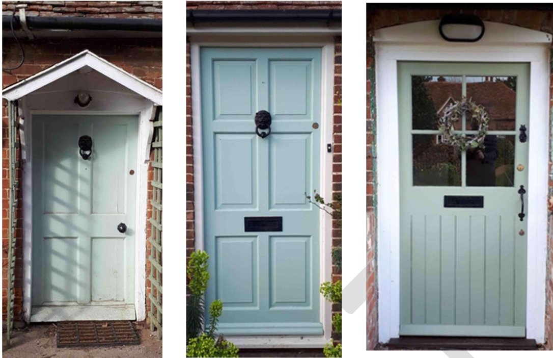
Figure 31: Examples of doors within the conservation area
