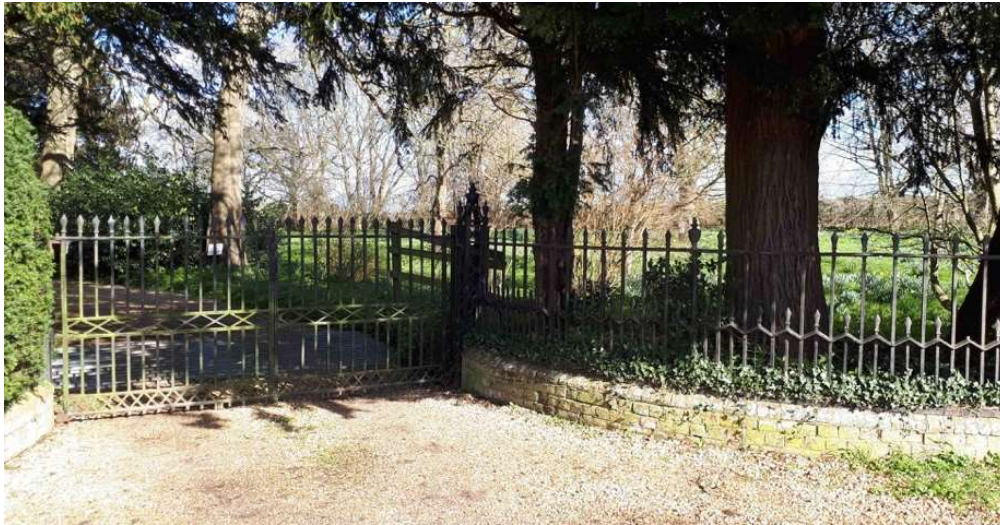
Figure 9: Listed cast iron railings at the entrance to The Old Vicarage.
