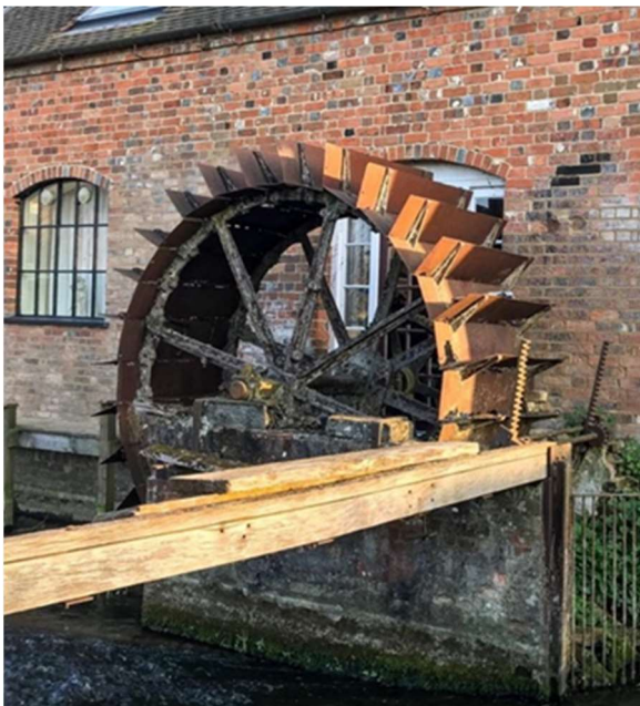
Figure 12: The water wheel that served the needs of the foundry
