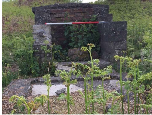
Plate 20 - concrete structure in quarry (19)
