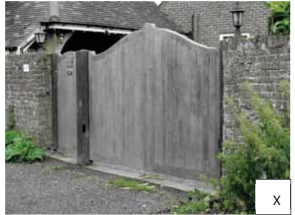
A high close boarded gate
