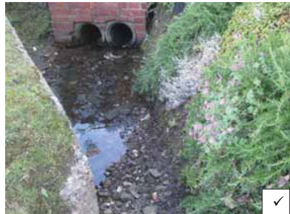
Well maintained ditch with planting on the bank
