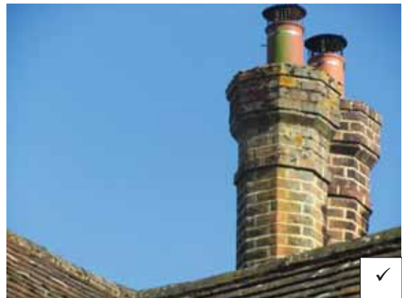
A decorative brick chimney
