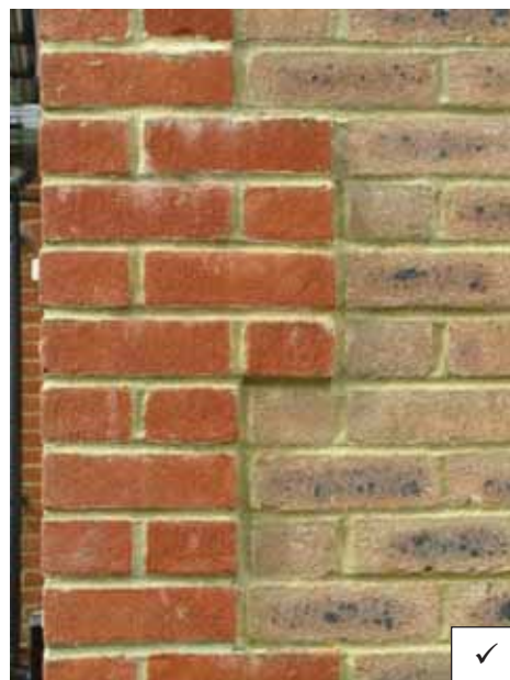
Contrasting quoins (corner stones)
