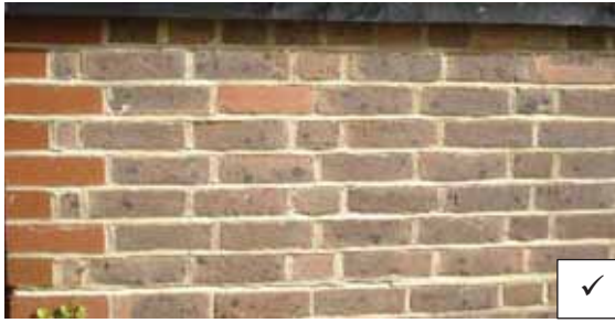
Another example of traditional laying using stretchers and headers
