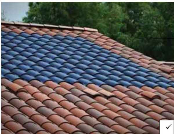
Solar tiles which contrast with the existing roof tiles
