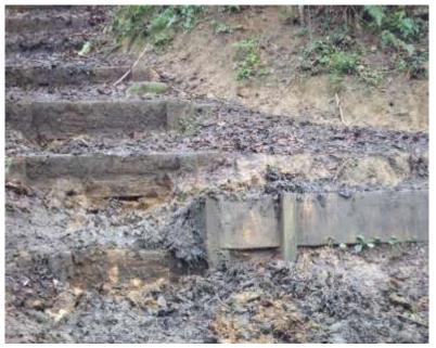
The main problem with the steps on the hill is the clay soil, which has poor drainage qualities and turns steps into a muddy, slippery mess.
