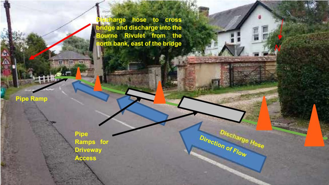
**Image E – The Vicarage and The Old Plough (beyond The Vicarage on left) – driveways to be provided with pipe ramps**
