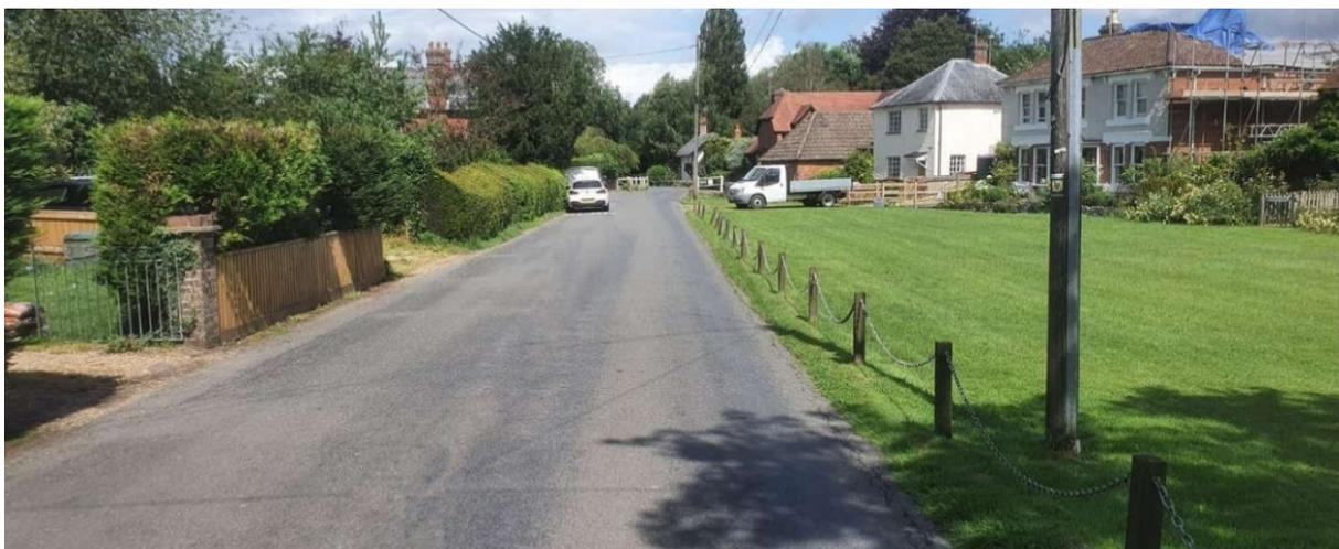
Figure 14 – Existing layout of B3046 and example with no centre line
