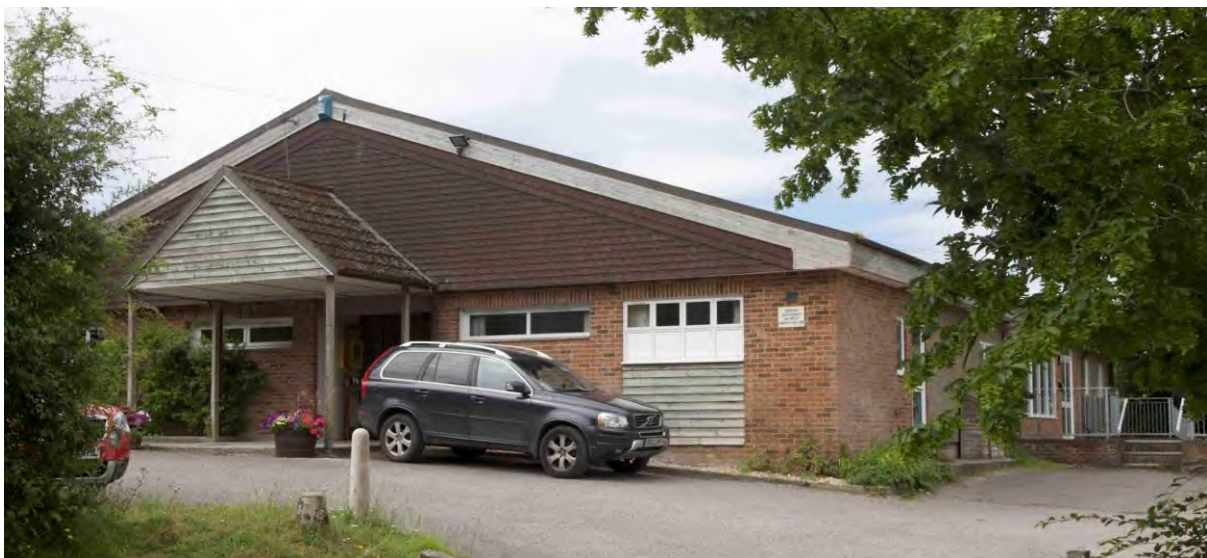
Figure 34: Coombe Bissett and Homington Village Hall, Coombe Bissett
